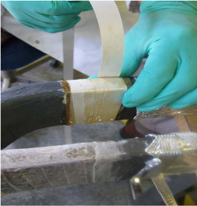
Figure 7.1 A coil that is in the process of being repaired after the coil insulation was accidentally crushed by a hammer blow just outside of the stator slot (Source: Courtesy Iris Power-Qualitrol).
