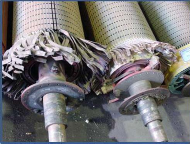
Figure 11.3 Two wound rotors in which the end winding banding has failed.
