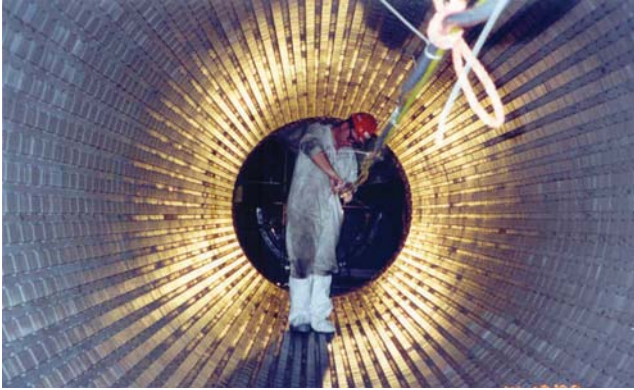
Figure 17.12 Excitation winding installed in center of turbine generator stator bore.
