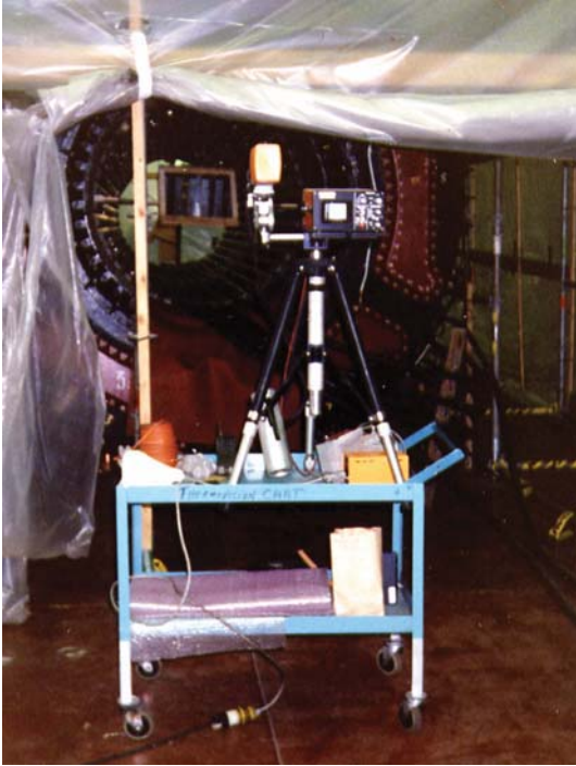
Figure 17.7 Thermal imaging camera and special mirror to monitor stator bore temperature in a turbine generator stator core.
