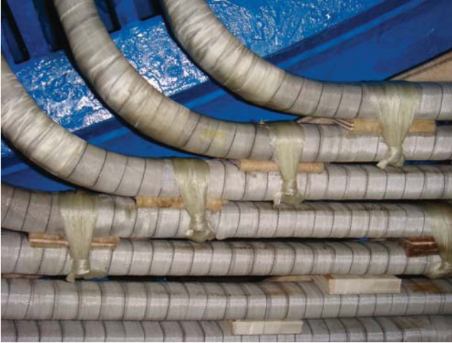
Figure 18.2 Butterfly ties at interbar blocking.
