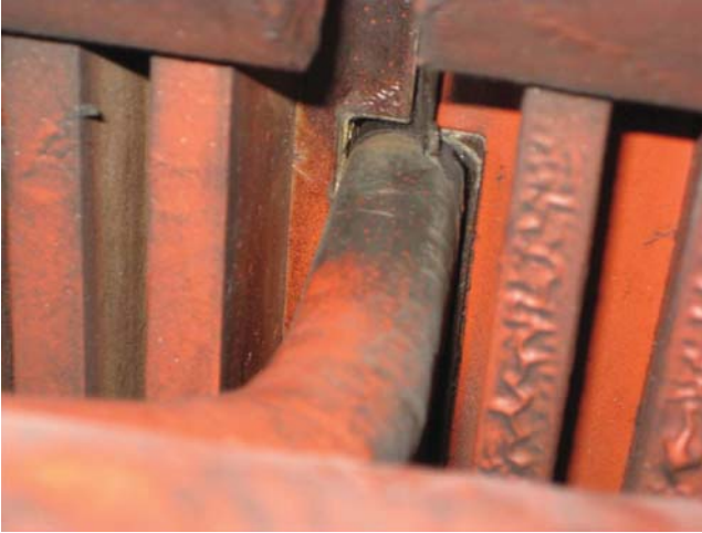
Figure 13.9 Split core packing movement.
